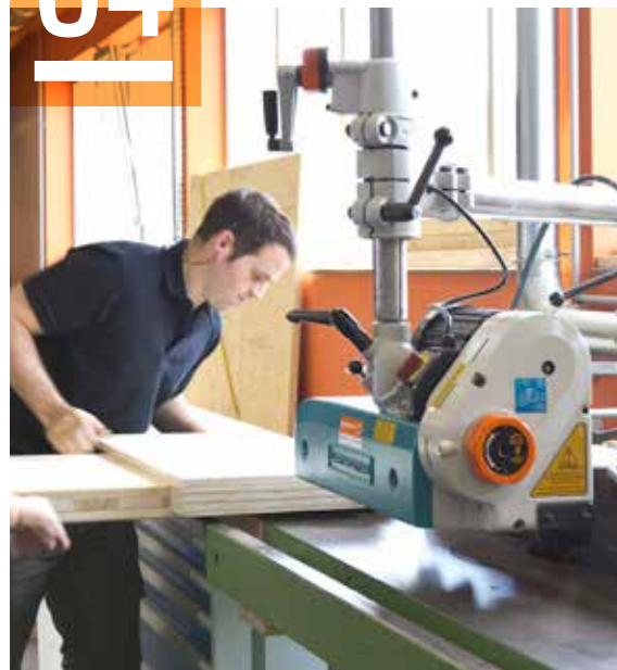
Cutting the infill elements from five-layer glulam.
